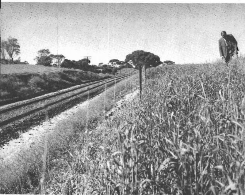
Previously threatened by drifting sand, the railway line is secure because of the stabilising grasses. Adjoining farmlands have been similarly stabilised and have returned to high productivity.
